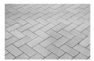
Block paving is built on a foundation.
